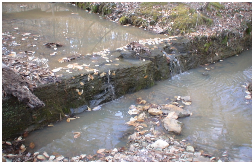
Figure 13: Example of grade control in Umstead State Park, Wake County NC (Susan Howard 2007).
